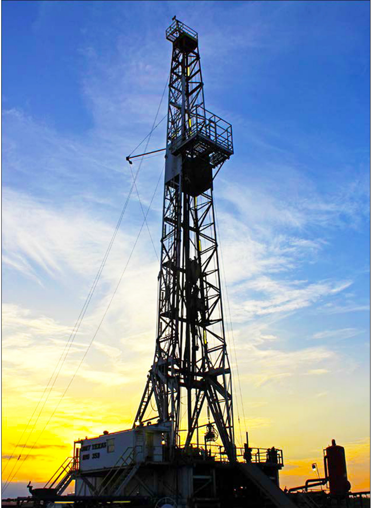
Figure 2. Unit Texas Drilling Rig #359 Drilling Holcomb 1-H
